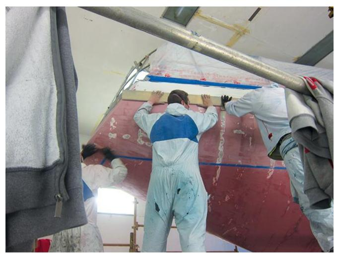
Shipwrights used templates from the line plan to build up and fair the hull
