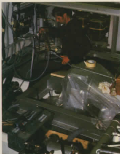
Order comes to electrical system chaos
