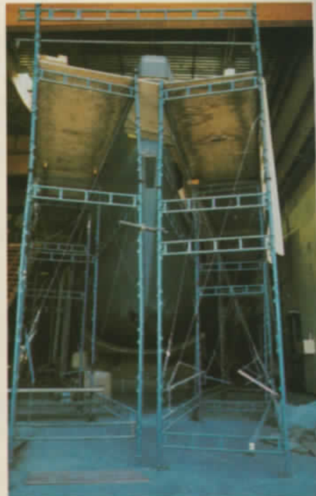
Two stories of scaffolding to the stemhead
