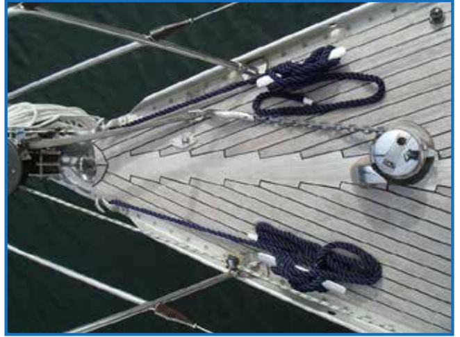
36 - Teack deck, with sharp batten corners
