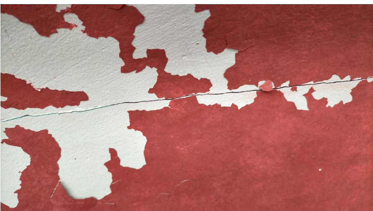
S&S Swan "smile", a thin crack between GRP hull and lead keel
