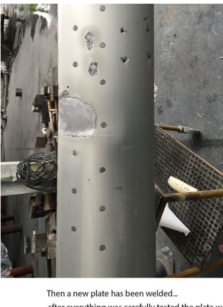
Then a new plate has been welded...
