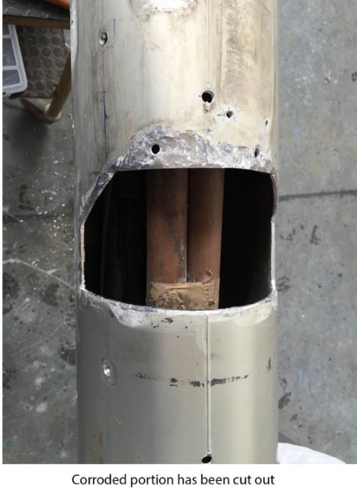
Corroded portion has been cut out
