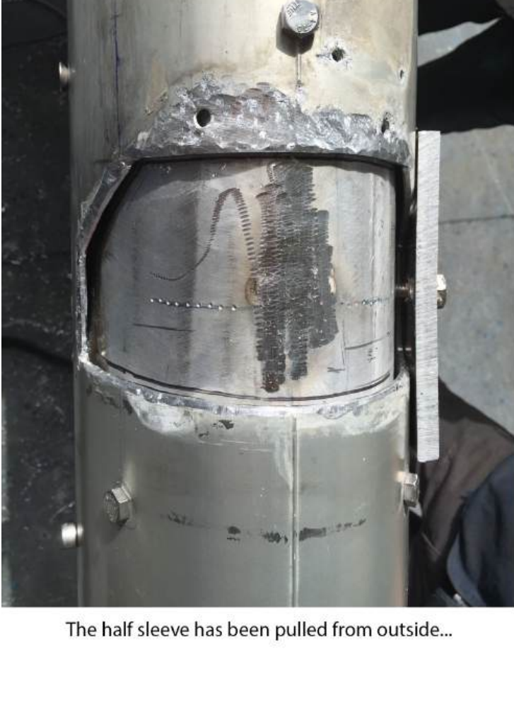
The half sleeve has been pulled from outside...
